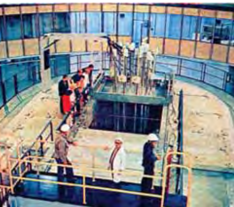
Construction of the Reactor Maria at the Institute of Nuclear Energy in Swierk, Poland.
