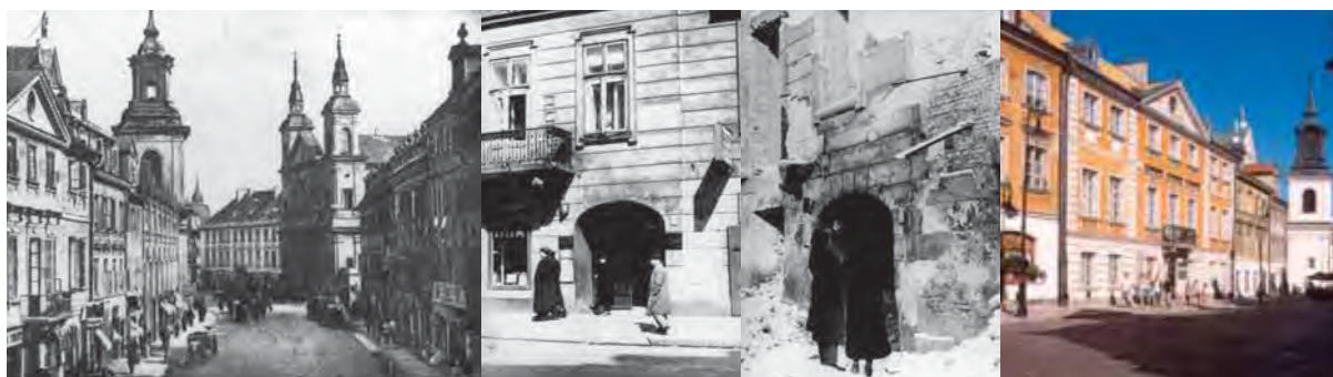
From left: Freta St. in the 19th century, the birthplace of Maria Skłodowska; 16 Freta St. in the 1930s; the building at 16 Freta St. was demolished during the Warsaw Uprising; the Maria Skłodowska-Curie Museum today.
